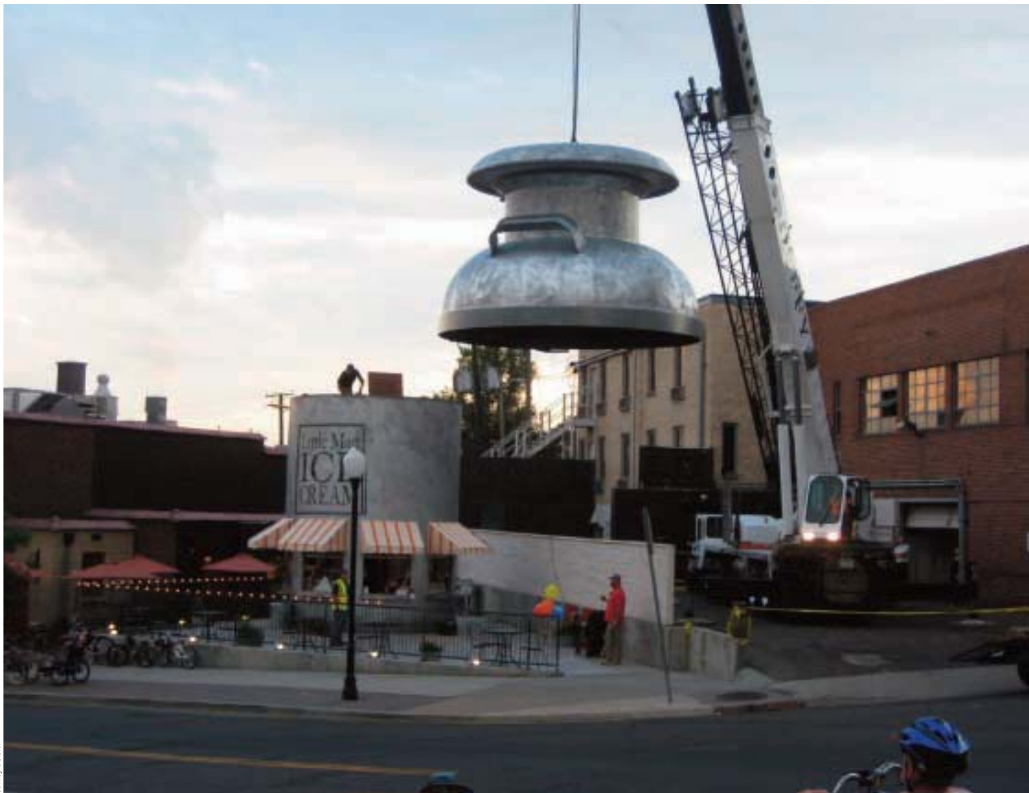
Above: The 6,000-pound cap was hoisted atop the cream can as part of the Little Man Ice Cream Grand Opening celebration. The architect designed the cap to be removable to allow the cream can to be transformed into a soup can with a ladle in the winter.
